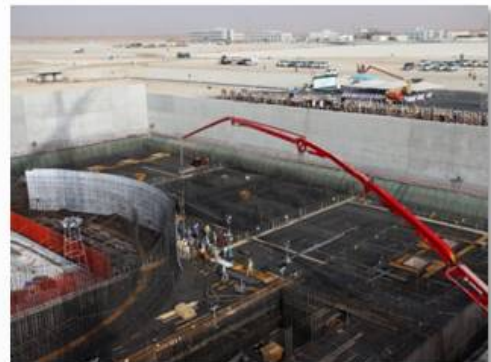
Reactor Unit 1 construction start July 2012, Barakah, Abu Dhabi, UAE
